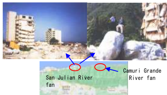
Fig. 6 Buildings damaged by debris flows on the San Julian River fan
