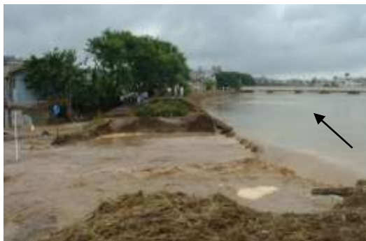
Photo 3 River bank breach at the Asuwa River, Fukui prefecture (Photo: Fukui Shinbun)
