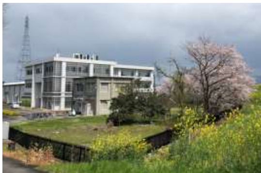
Photo 5 New research building of the Research Center for Fluvial and Coastal Disasters, completed in Dec. 2013
