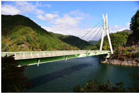
Figure 1. A side view of investigated bridge
