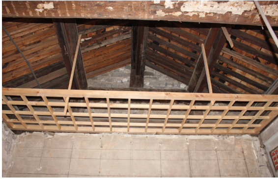
Figure18 The traditional suspended ceiling of siheyua
