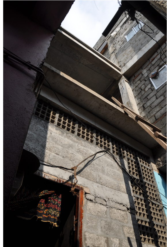
Figure 20 The New Structure Stands with Support from the Existing Structure: The Nucleus of the Physical Common Support
