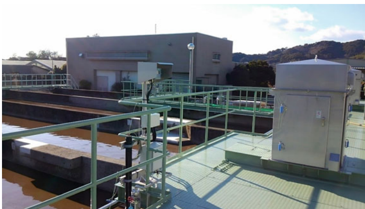
Fig. 11.1 Oxidation ditch at Yasu WWTP, Konan, Japan. (Photo: provided by Maezawa Industries, Inc.)
