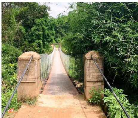
Figure 3. The bridge built by the Had Yao Rubber Cooperative
