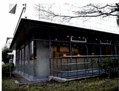
Wa-on (East side of Jinkan building)
