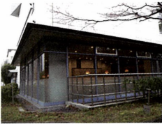
Wa-on (East side of Jinkan building)
