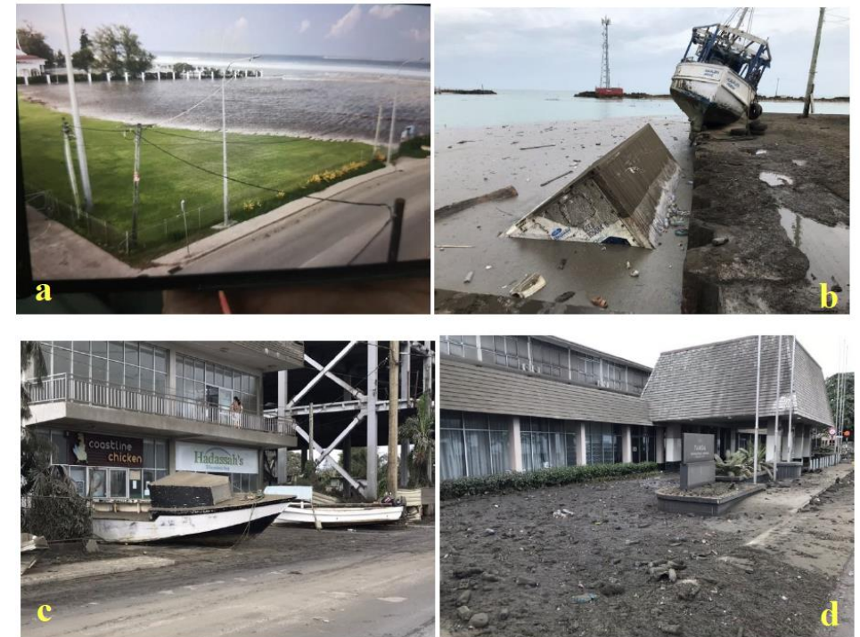
Fig. 10 Scenes from Nuku'alofa (a) tsunami surge coming on the grounds of the Royal Palace at 17:47 local time (b, c) some smaller vessels were floated on to the wharf decks (d) inundation at the Tanoa Hotel along the waterfront.
