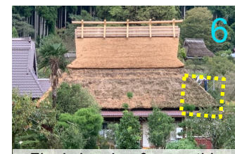
Final cleaning & smoothing
