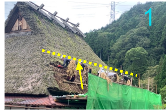
Removal of old thatch
