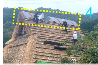
Placement of metal sheets
