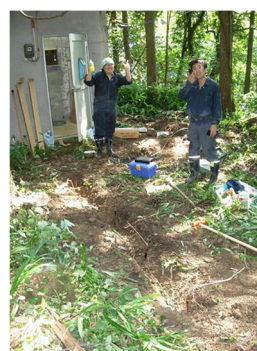
Photo. 7 Class A grounding work
