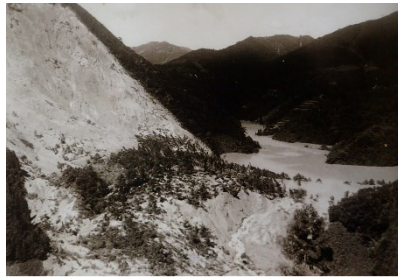
B: Landslide dam of Kongouji landslide
