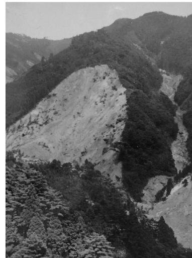
F: Arinaka C landslide
