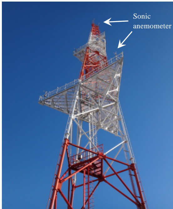
Photo 1 Observation tower in the Ujigawa Open Laboratory. Sonic anemometers at 55 m and 25 m are indicated
