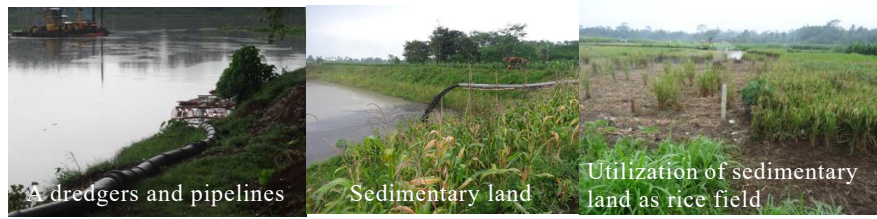
Photo 8 Dredging in Sutami Reservoir in the Brantus River
