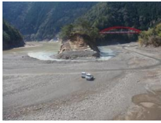
Photo 11 Sediment deposition at the upstream end of Futatsuno Dam in Kumano river due to Typhoon Talas in 2011 Peninsula
