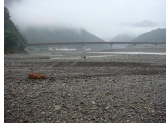
Photo 11 Sediment deposition at the upstream end of Futatsuno Dam in Kumano river due to Typhoon Talas in 2011 Peninsula
