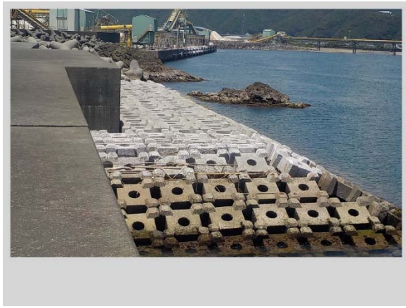
Photo 12 Counter-weight mound in Suzaki breakwater
