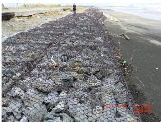
Photo 8 Wave dissipating later to prevent scouring
