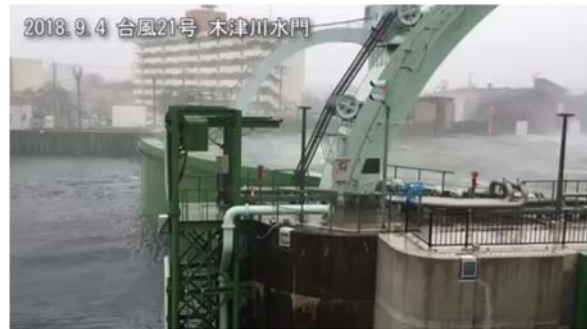
Photo 14 Protection of storm surge generated by typhoon No.1821.
