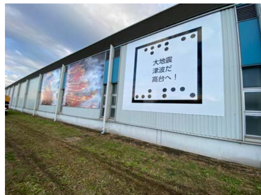
Photo 10 Installed two signboards and one AR signboard
