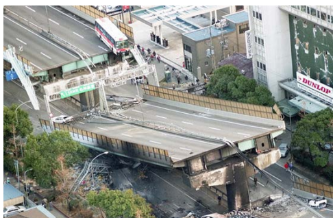
Photo 1 Example of damages caused by the Great Hanshin-Awaji Earthquake in 1995 ( https://www.bosai.yomiuri.co.jp/feature/4664 )
