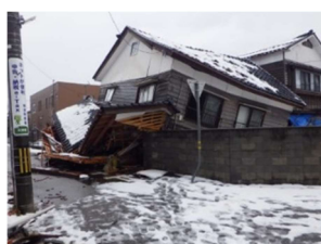
Photo 2-15 Heavily damaged wooden house
