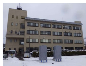
Photo 2-9 Wajima Regional Joint Government Building
