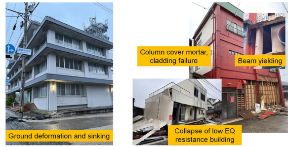
(a) RC building
