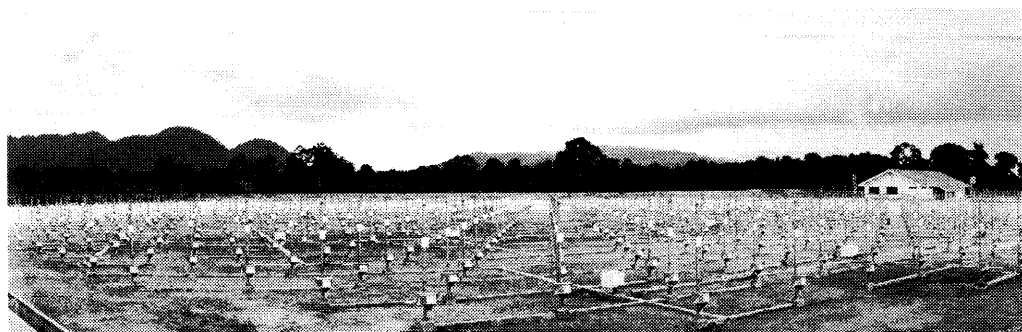
Figure 1: Picture of EAR installed at Koto Tabang, West Sumatra, Indonesia
