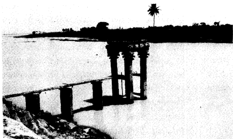
Plate 4 Sluice at the Hoskote Reservoir. Note the stone slabs placed on brick-built columns which provide access to the sluice from the embankment.
