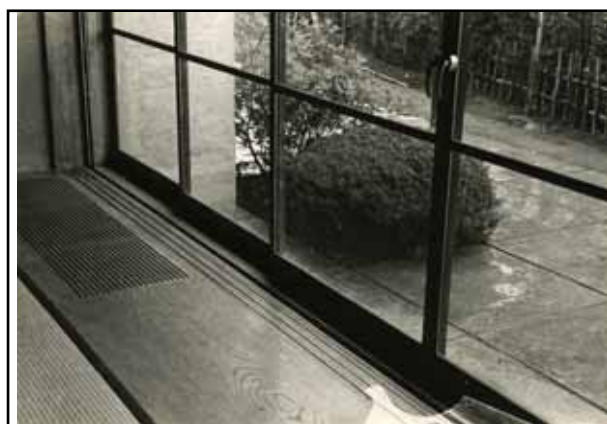
Sliding doors in Japanese room with floor heating grid on the left (1F)
