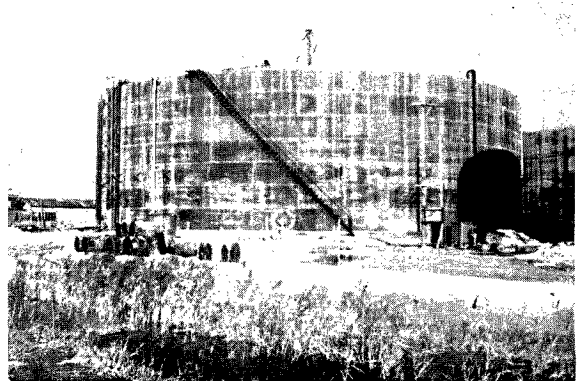
Fig. 12 Front view of oil tank
