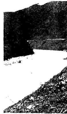
Photo 7. A view of the section No. 6 during unusual low water level in sept. 11, 1965.
