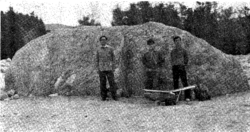
Photo. 3 A radio-controlled model aeroplane for the special photo survey and a large concrete block (10m×2m×4m) which flowed down in the distance of 800m along the valley from the broken dam. This large block is looked in Photo. 2.
