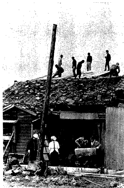
Photo. 4 Damage to a wooden house. (Courtesy the Mainich-shimbun)
