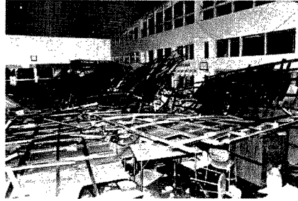
Photo. 5 Damage to a steel structure. Complete removal of the roof and collapse of the ceiling (Tsuboya). (Courtesy the Chunichi-shimbun)
