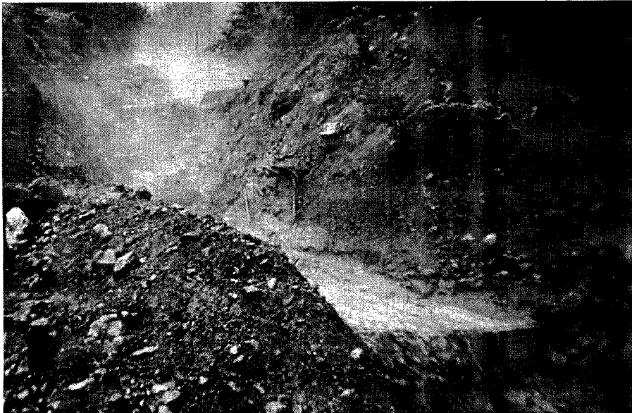
Photo. 8 Muddy stream flowing over dam No. 6 (lower dam) immediately after passing of mudflow front.
