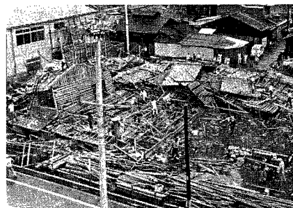
Photo. 11 Collapse of ten wooden houses in construction, KYOTO (by the courtesy of the Kyoto Shimbun).
