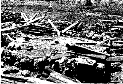
Photo. 1 Ruins of a blown-off house, Zaha, OKINAWA.
