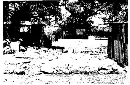
Photo. 6 Ruins of a blown-away house, Komesu, OKINAWA.
