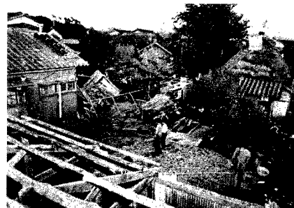
Photo. 3 Damage to structures.
