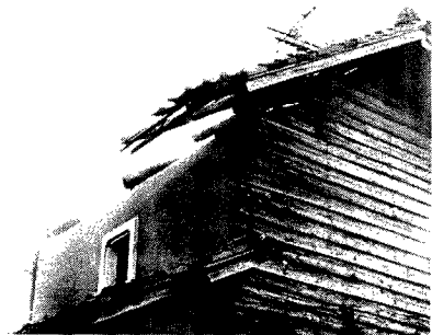
Photo. 2 Damage to a wooden house.
