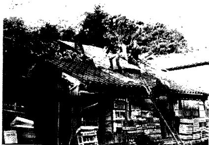
Photo. 4 Local damage to a wooden house.
