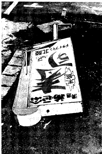
Photo. 6 Damage to the sign tower (1).
