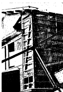
Photo. 3. Damage to external wall: wooden house.
