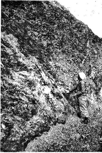
Photo. 3. The fracture zone in the landslide area.
