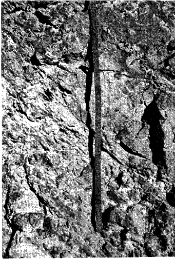
Photo. 7. Weathered sandstone in the landslide area.
