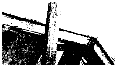
Photo. 8. Detail of a damaged beam and column.
