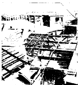
Photo. 6. Roof failures due to uplift in Serica.
