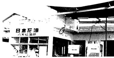
Photo. 22. Roof failure due to uplift.
