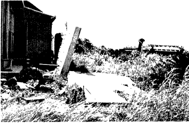
Photo. 23. Failure of concrete block fence.
