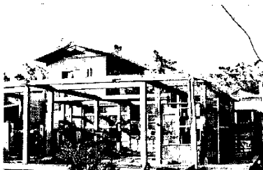
Photo. 5. A completely damaged house in Kuranuki.
