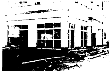
Photo. 18. Damage to glass panes in Tamina.
