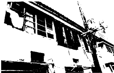
Photo. 10. Damages to the wooden window frame.
