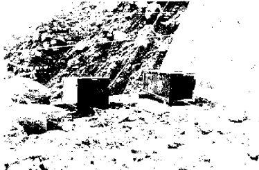
Photo. 2. Debris samplers set on a Sabo-dam.
