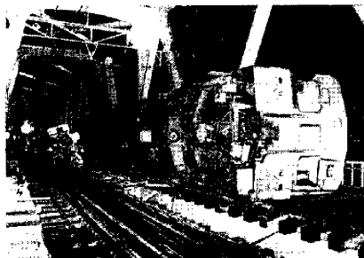
Photo. 1. Derailment of a train shown in Fig. 14.
