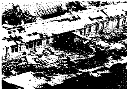
Photo. 2. Damage to a prefabricated school building shown in Fig. 15.
