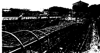
Photo. 1. Damage to a vinyl plastic greenhouse. Its position is pointed A in Fig. 6.
