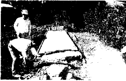
Photo. 2. Damage to a concrete block fence.
