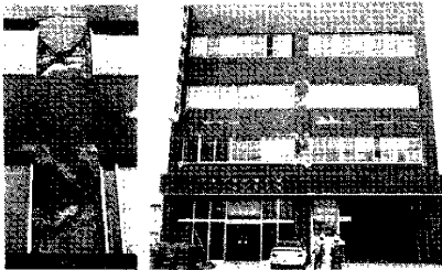
Photo. 25. Whole view of B-building and shear failure of columns.
