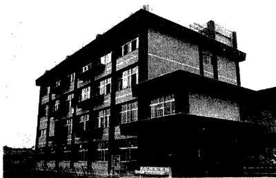
Photo. 1 Example of B-type school building (Hachihonmatsu primary school).
