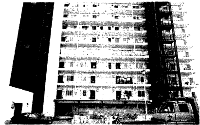
Photo. 33. Damage of non-structural walls in apartment building.
