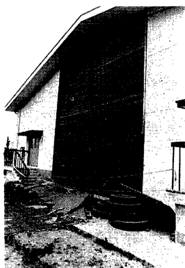
Photo. 4. Damage of walls (Daiwa primary school).
