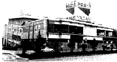
Photo. 10. Example of damaged reinforced concrete buildings.
