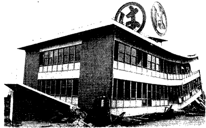
Photo. 8. Example of damaged reinforced concrete buildings.
