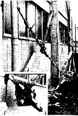
Photo. 32. Breakage of braces.
