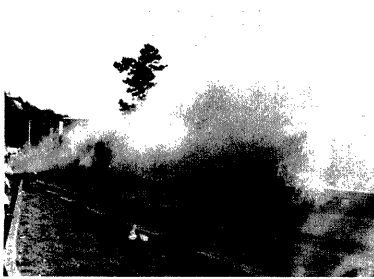
Photo.2 Wave overtopping by Typhoon 7920 at Nishihama coast.
