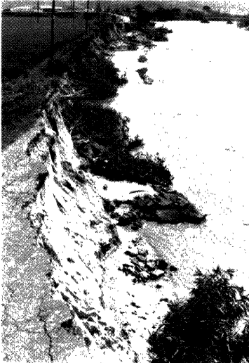
Photo. 5 Bank erosion and flood fighting works by bamboo grass near Ishizue Bridge looking downstream.
