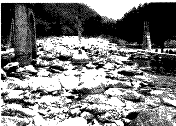
Photo. 1 Yokitogi Bridge looking upstream.
