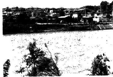
Photo. 6 Bank erosion close to the residential area downstream Inazu Bridge (1.0 km). (downstream to the left)
