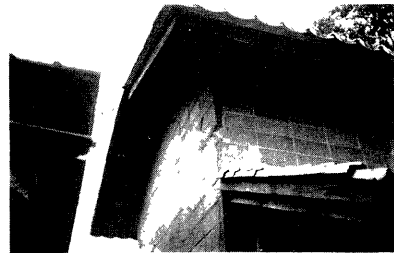
Photo 4 Cracks in concrete block wall
