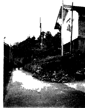
Photo 2 Failure of banking soil
