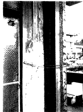
Photo 12 Shear failure of a reinforced concrete column
