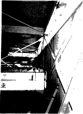
Photo 7 Buckling of steel braces
