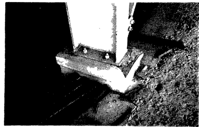
Photo 6 Damage at column base
