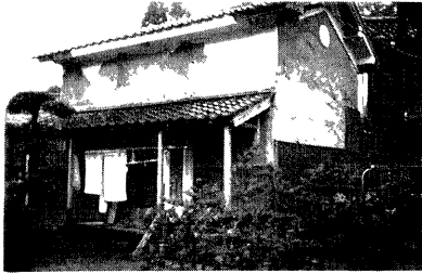
Photo 1 Falling down of wall finishing
