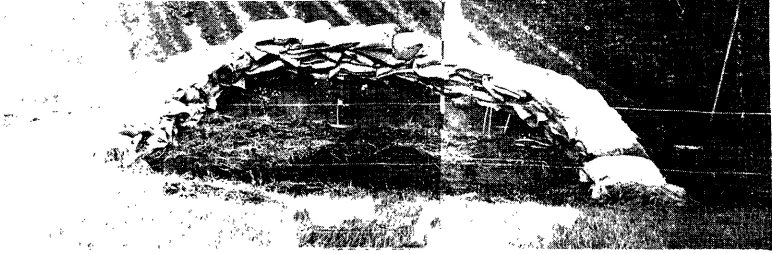
Photo 6 Tsukinowa-ko (semi-circular hooping by sandbags to store leaking water and reduce the seeping water pressure) in the Chikuma River (after a flood)
