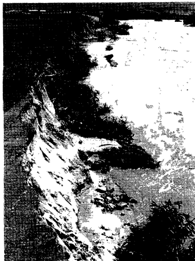
Photo 5 Takenagashi-ko (bank erosion protection by bamboo grass) in the Daido River (during a flood)
