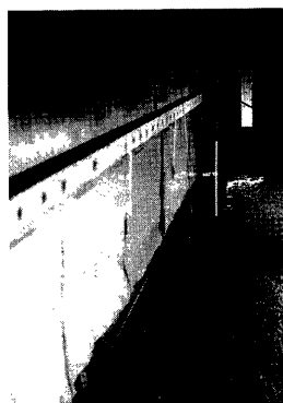
(a) Looking downstream
