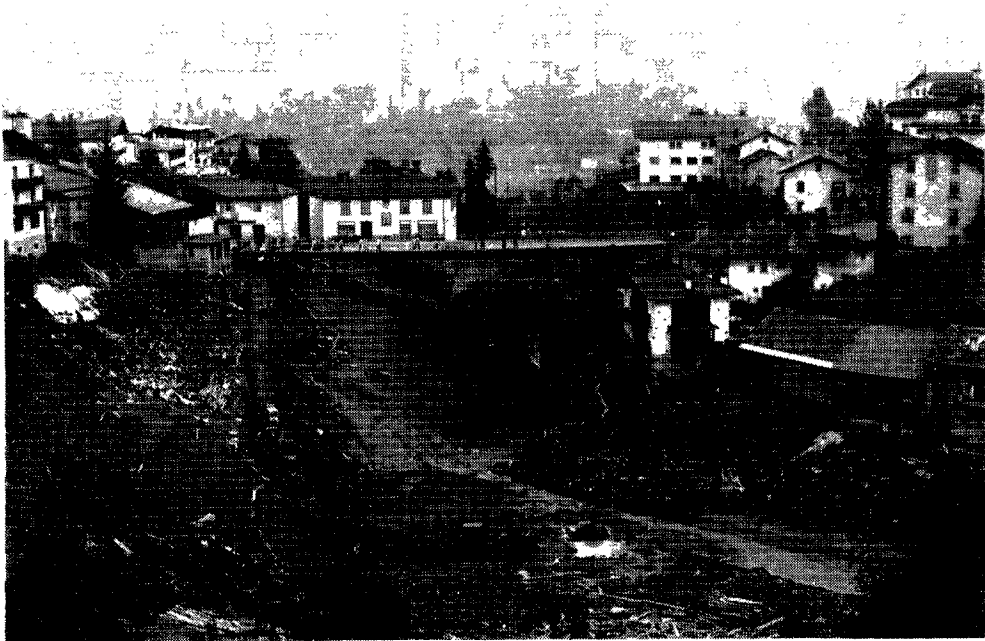
Photo. 11*. Romano bridge and upstream after the mud flow.
