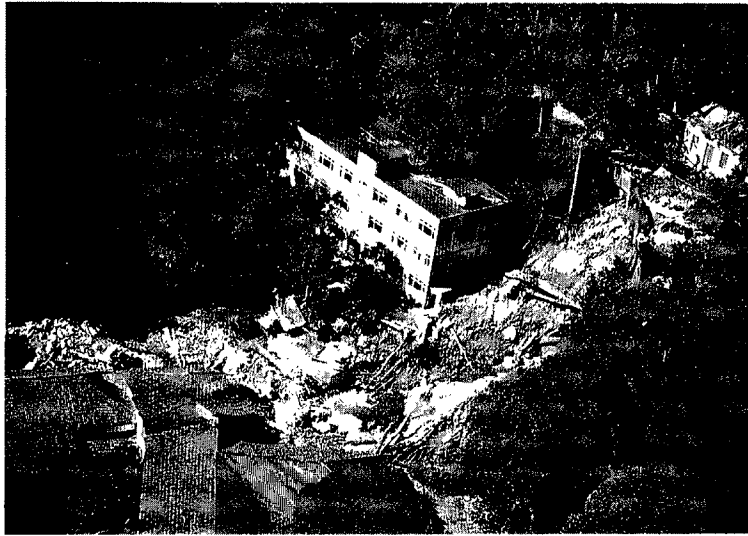
Photo 8 Debris flow with many large rocks of 500 tons in total attacked Santa Jenoveva hospital and 40 persons died.
