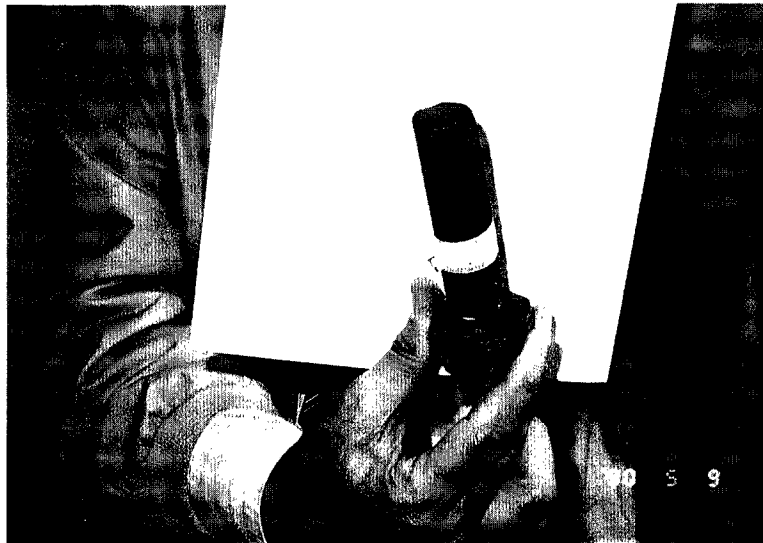
Photo. 18. One-inch anchor bolt sheared off on Pier E9 of Bay Bridge (photographed at UC Berkeley, Prof. A. Astaneh's Lab.).
