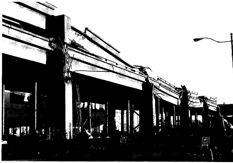
Photo. 23. Collapsed I 880 Cypress St. Viaduct-III (Type II; photographed on 11/4/89).
