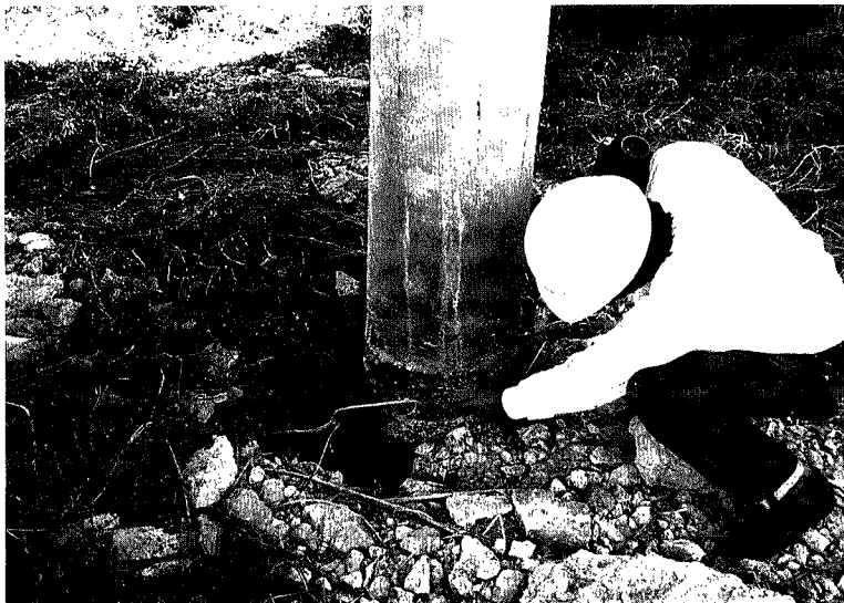
Photo. 25. Dislocation of a pile bent of Struve Slough Bridge (photographed on 11/5/89).
