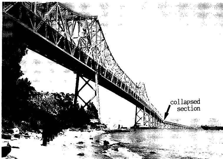
Photo. 17. Truss sections of the Oakland side of Bay Bridge.
