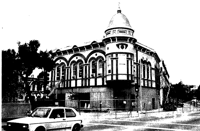
Photo. 11. Leonard Building in Santa Cruz damaged by the Loma Prieta Earthquake.
