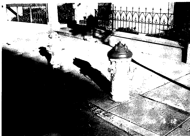
Photo. 28. AWSS hydrant (right) and MWSS hydrant (left).
