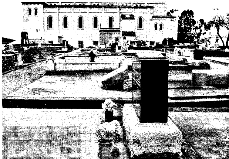
Photo. 2. Tomb stones dislocated and/or turned-over during the Loma Prieta Earthquake (St. Francis Cemetery near Watsonville; photographed on 11/5/89).
