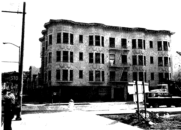
Photo 9. Apartment building (same as the one in Photo. 7) under repair works (photographed on 5/13/90).
