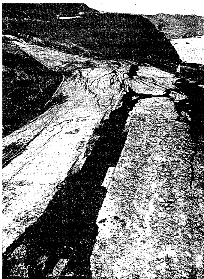
Photo. 4. Section of Hwy. 1 affected by slope failure near Muir Beach 22) .
