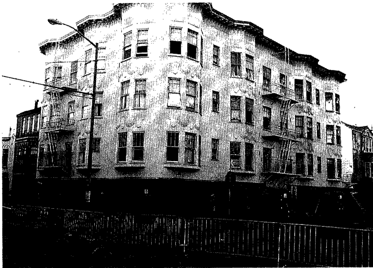
Photo. 7. Failure of a wooden apartment building in Marina District of San Francisco (photographed on 11/10/89).
