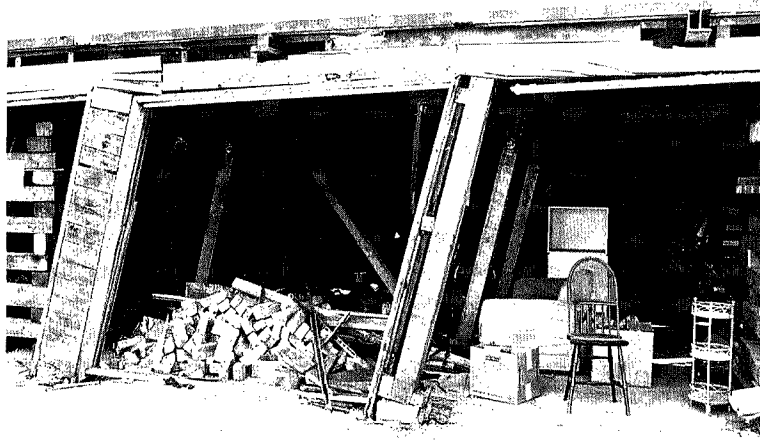
Photo 8. Failure of soft first storey of an apartment building in Marina District (photographed on 11/10/89).
