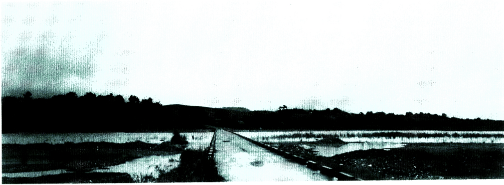
Photo 21 Bato Ferry submerged bridge.
