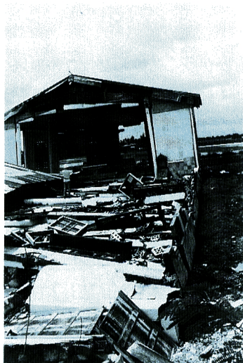
Photo 10 A church collapsed by liquefaction at Pura.
