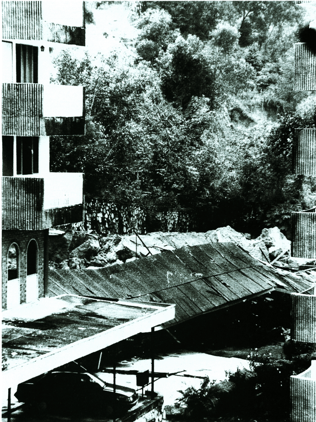
Photo 1 Starting landslide behind the building.
