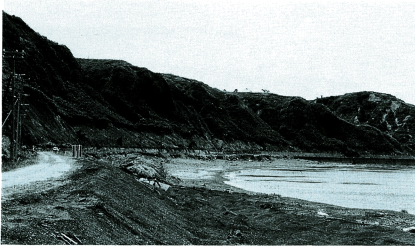
Photo 9 Marks of tsunami runup on a hill slope along Aonae-Monai coast (the height is about 10m above M. S. L.).
