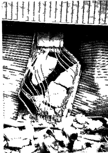
Photo 11 Shear failure of the first story column.
