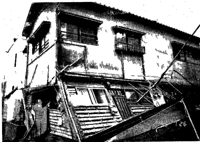
Photo 3 Collapse of inner-connected wood apartmenthouse.
