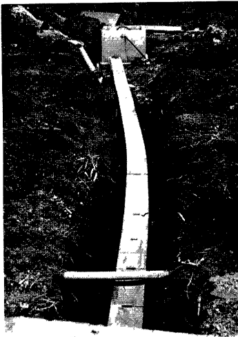
Photo 2 U-shaped concrete covers in which a water-tube and an air-tube are set.
