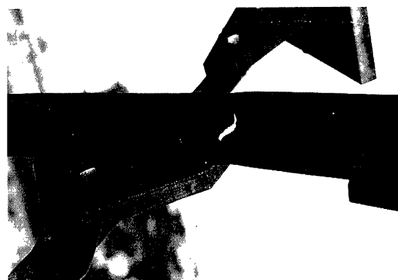
Photo. 14. Rupture of an angle brace.
