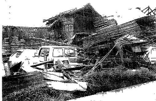
Photo. 3. Completely Destroyed workshop of car maintenance (Ohmisaki, Kushimoto).
